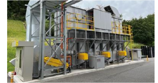
Installation of energy-saving equipment (Koka City, Shiga Pref.)
